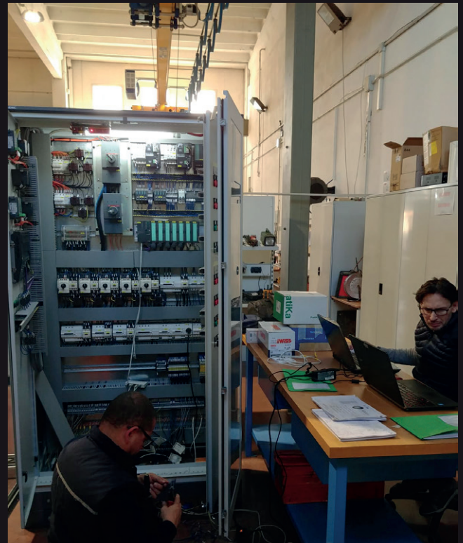
PLC SIEMENS 1514 - OPTICAL FIBER
